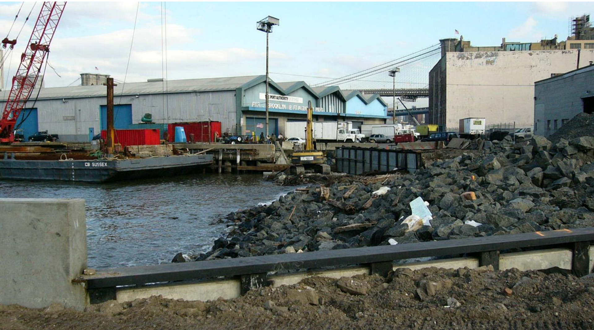
Brooklyn waterfront, before restoration
